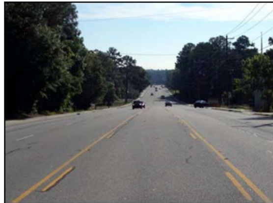
In comparison, the 5-lane segment of Platt Springs Road has no visual clues to the drivers that vehicle speeds should be reduced.
